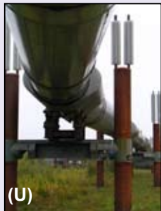
(U) Trans-Alaskan Pipeline
