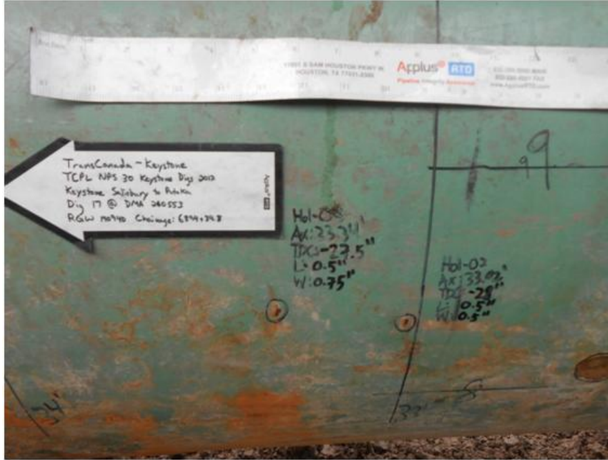
Figure 25. MP1000.32 – External Corrosion Pitting
