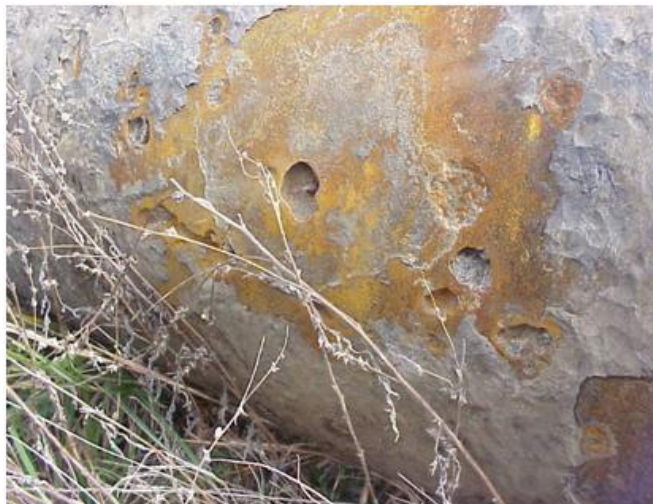
Figure 5. Typical D-C Stray Current Corrosion Morphology
