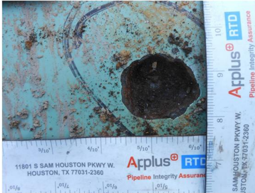
Figure 13. MP 996.33 –External Corrosion Pitting
