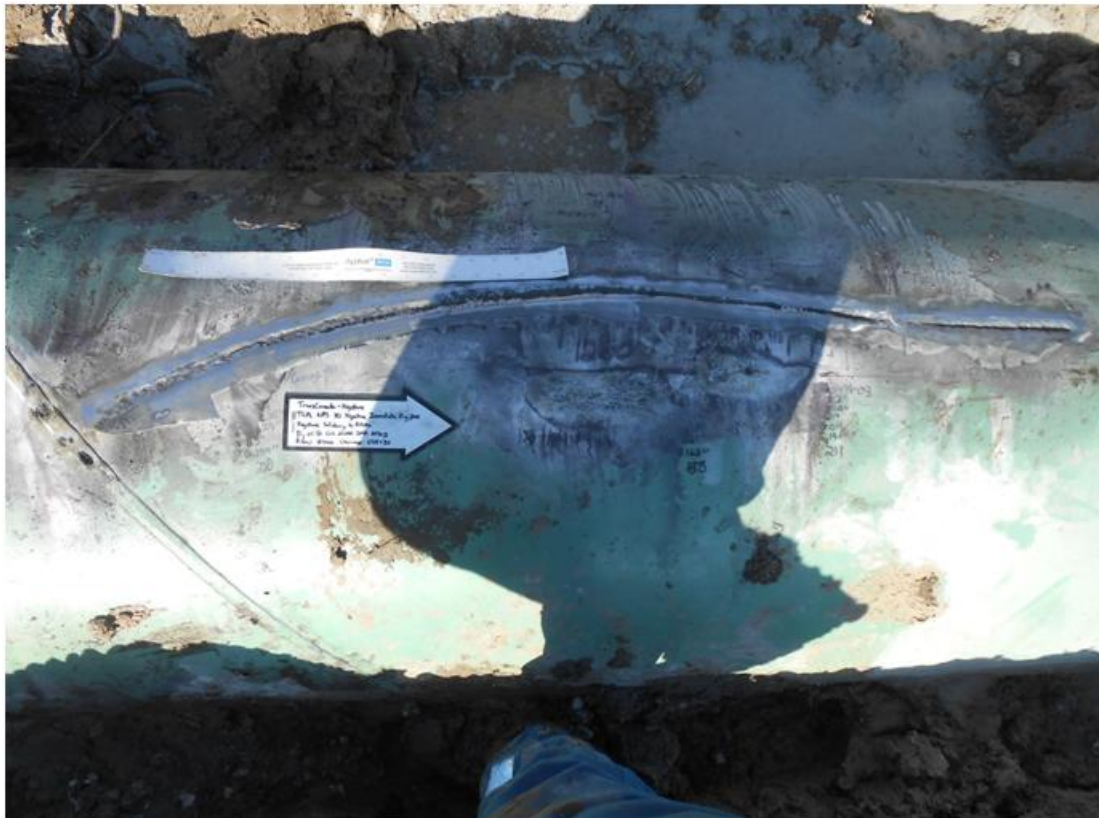
Figure 18. MP 997.67 – Axially Oriented External Corrosion at Areas of Coating Damage
