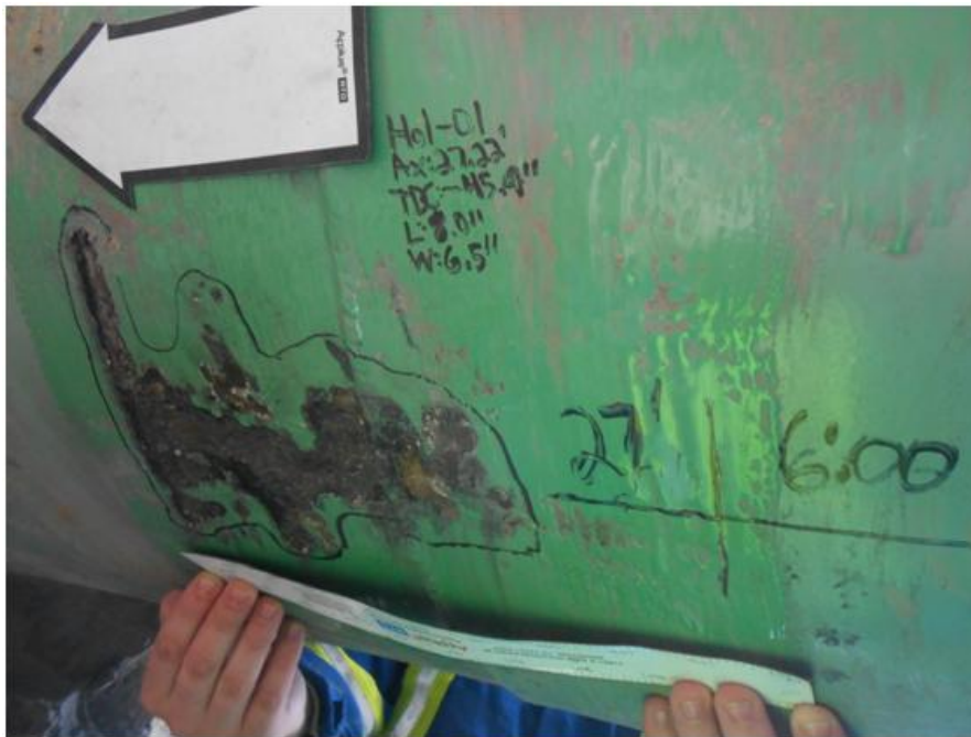
Figure 23. MP 999.97 – Coating Damage
