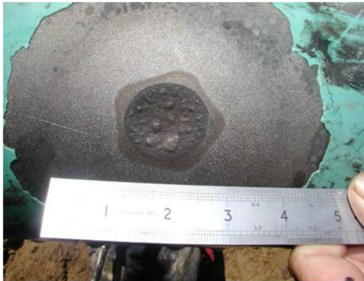
Figure 6. Typical A-C Corrosion Morphology
