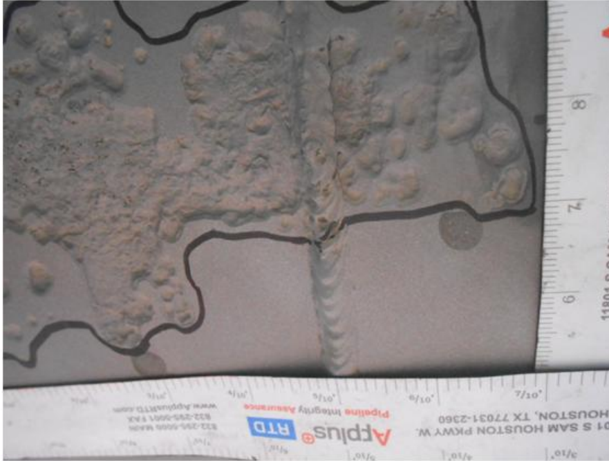
Figure 24. MP 999.97 – External Corrosion
